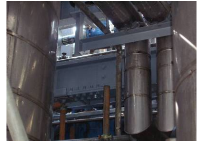
Inspection revealed corrosion treatment and replacement of some I beams required
