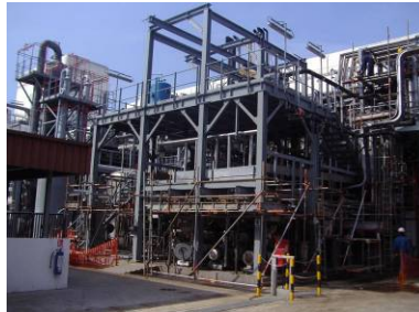
Inspection revealed corrosion treatment and replacement of some I beams required
